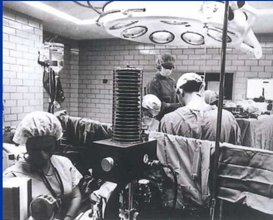
FIGURE 5. Operating room in the original hospital (now rooms 14-18)
