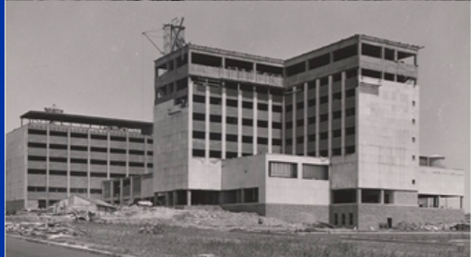
FIGURE 2. Construction of the new Medical Center
